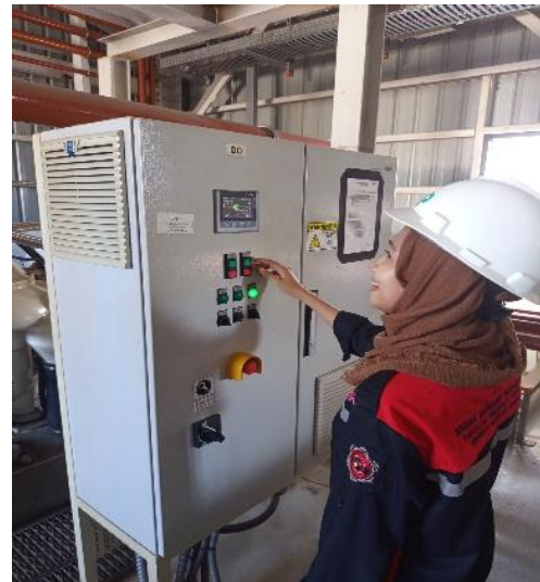
Gambar 4, Pengoperasian kontrol sistem Diesel Oil Separator (DOS)
